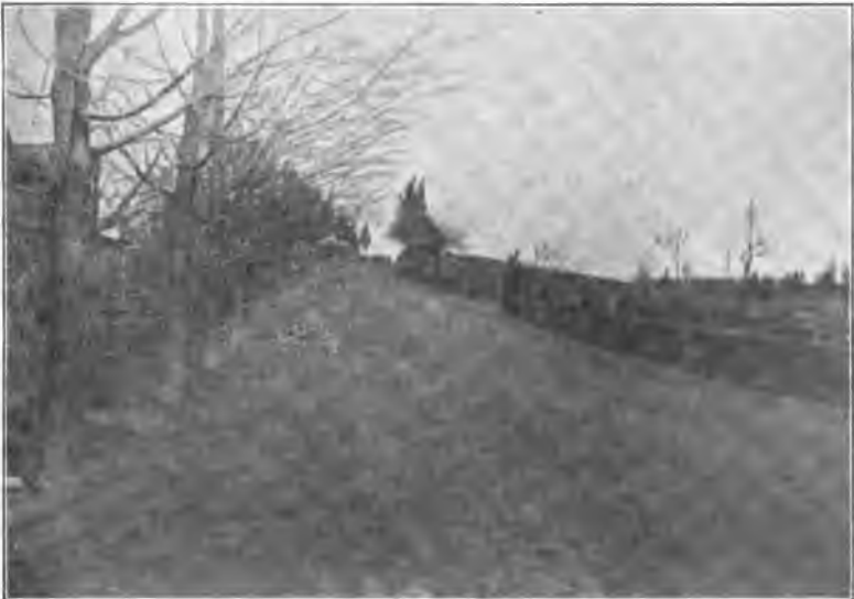
Squaw Brook road, Passaic Co., after improvement.
